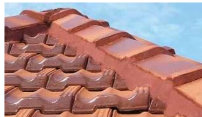
8. ROOF POINTING Pointing is a flexible material that covers mortar and matches roof tile colour. Roof Pointing helps keep the ridge in strong and intact.
