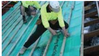
4. NEW BATTENS INSTALLED Before laying roof tiles, new battens are installed.
